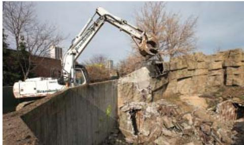
Brandenburg utilized track excavators equipped with multiple attachments, and skid steer loaders to demolish and process the building, slabs, foundations and walls.
