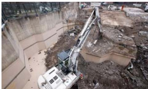
All concrete removed during demolition was crushed to three inches minus and the material was used as backfill onsite. All demolition debris was recycled, removed or disposed from the site in accordance with all applicable local, state and federal guidelines.
